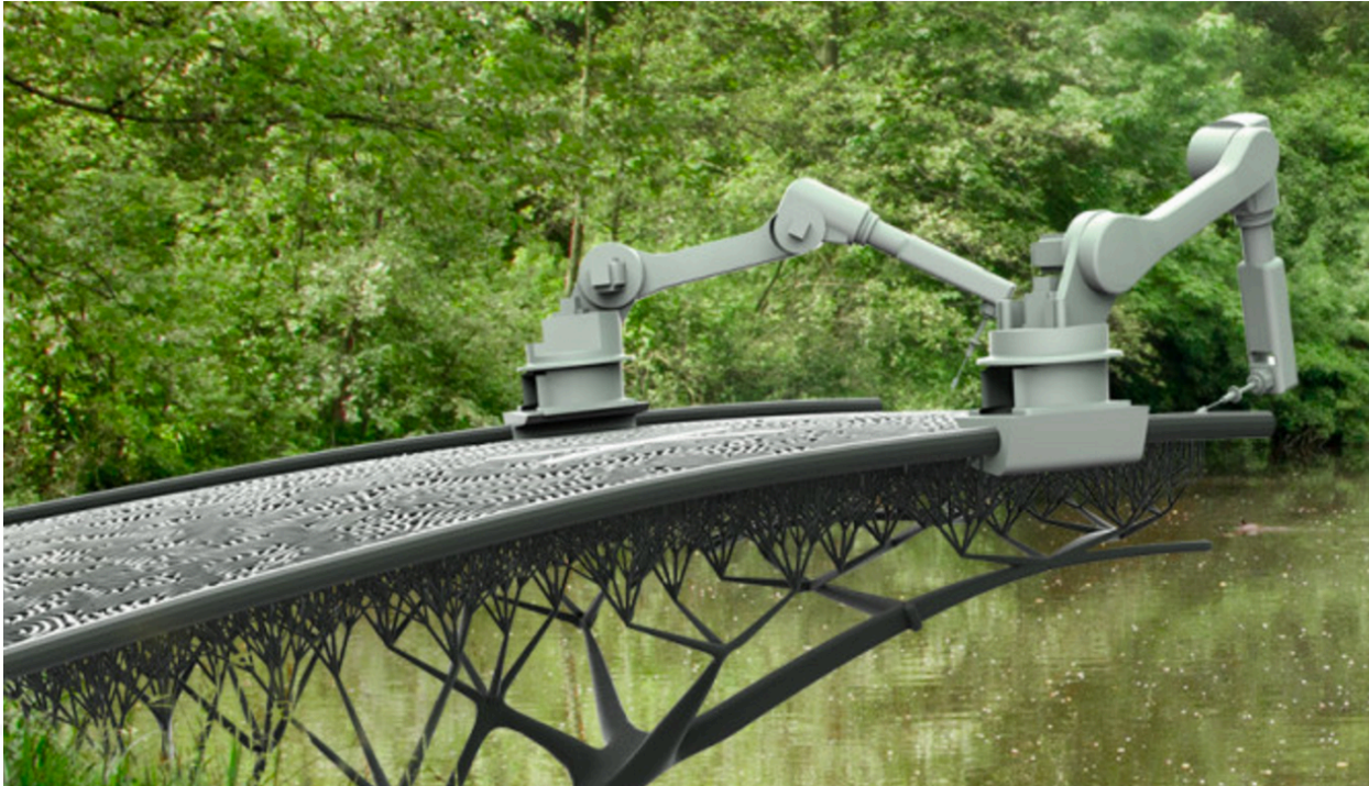
MX3D Bridge – 3D printing a steel bridge in Amsterdam
